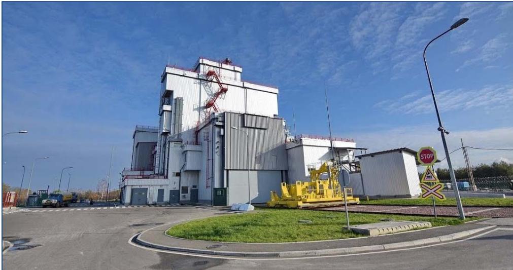
Figure 44: Completed Processing Facility of the Interim Spent Fuel Storage Facility 2
