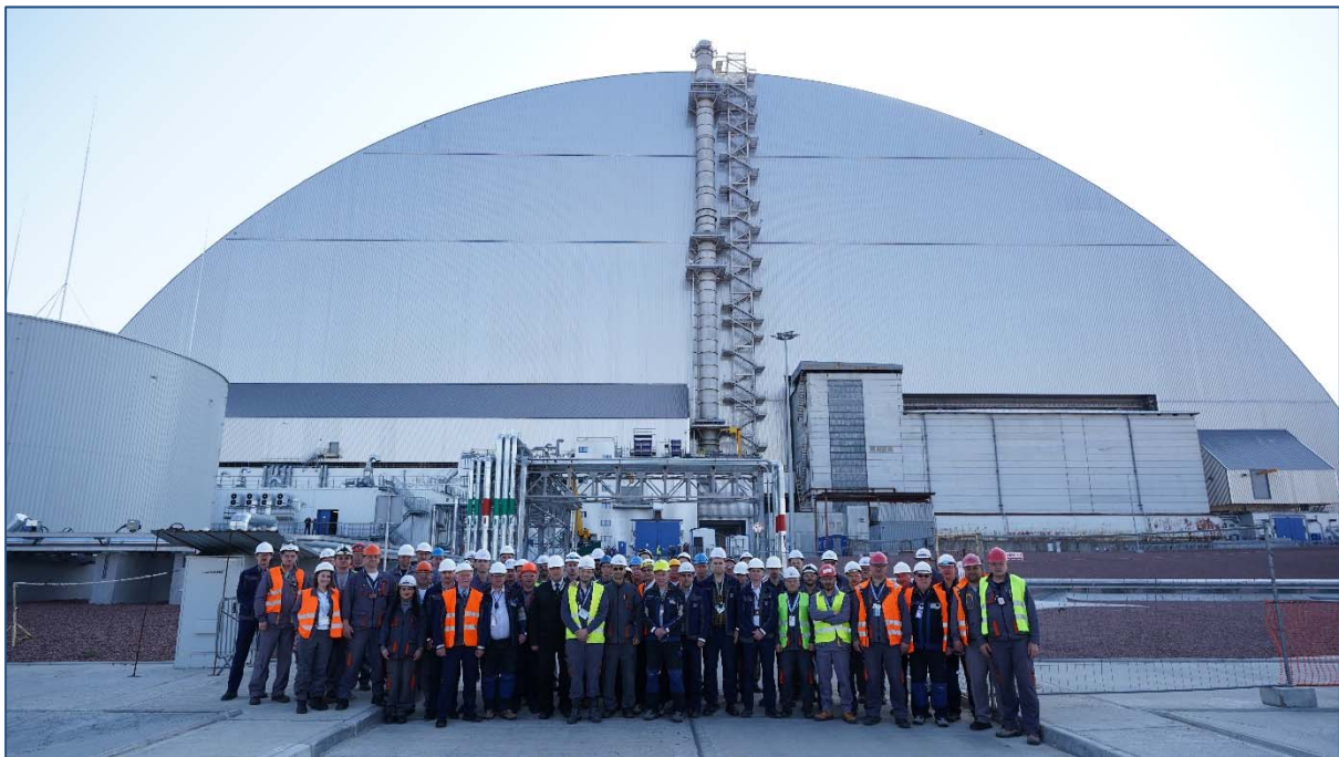
Figure 43: Completed Chernobyl New Safe Confinement in April 2019
