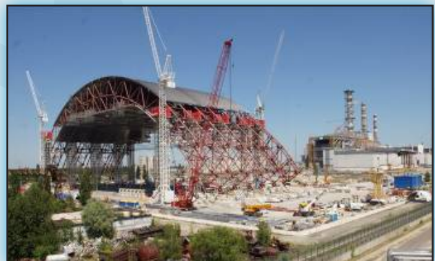
Second jacking stages of the Arch east part
