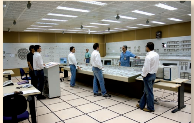
Angra-2, Brazil (Photo: Eletronuclear, Brazil)
