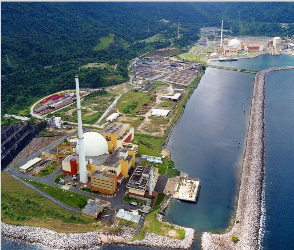
ANGRA-3 nuclear power plant, Brazil (Photo: Eletronuclear, Brazil)
