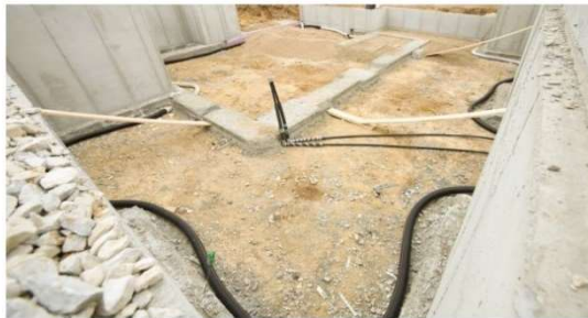
A radon mitigation system in the basement of a house. The EPA is calling on people in high radon areas to test their homes for the gas. File photograph: iStock
