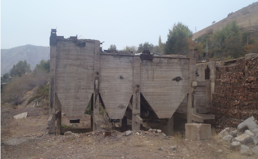
Abandoned infrastructure in Yangiabad.
