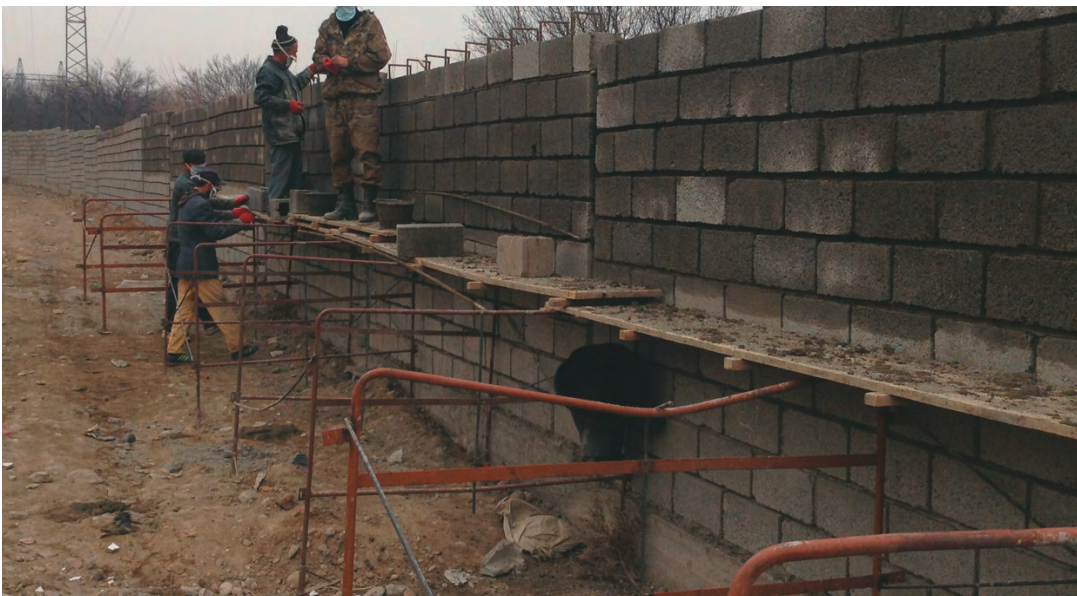
Construction of the concrete wall around Karta 1-9.
