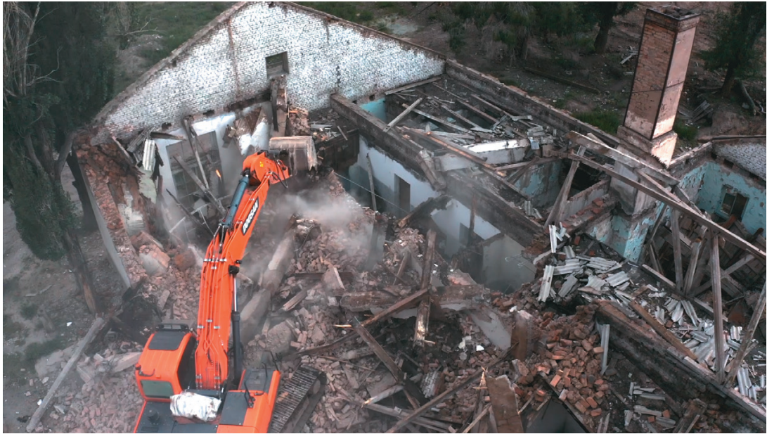
Demolishing of building infrastructure in Min-Kush under the ERA Programme
