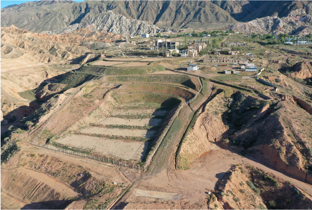
Tailing dump in Kadji-Sai village, after remediation, September 2020.
