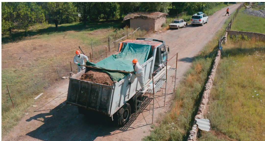
Transport of waste material from Shekaftar to remote waste repository.
