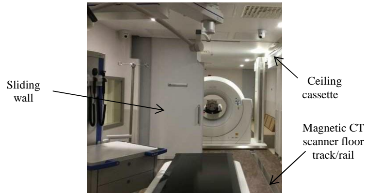
FIG. 2. Sliding wall between the CT Room & Resus Room (view from Resus Room).
