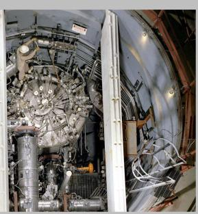
Typical nuclear reactors (light water reactors) use solid uranium oxide fuel, with liquid water as their coolant and moderator.
