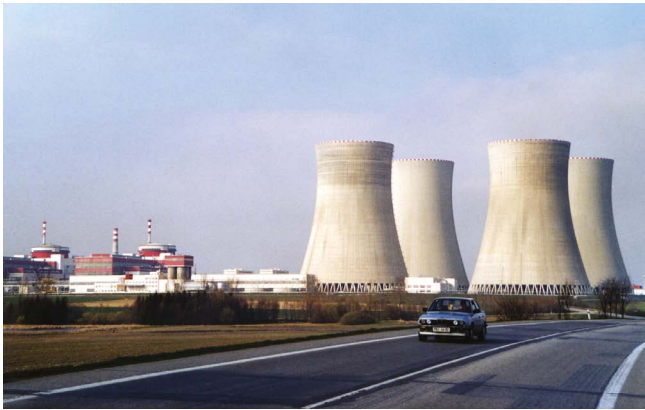
The Temelin Nuclear Power Plant in the Czech Republic (Photo: Vadim Mouchkin/IAEA)
