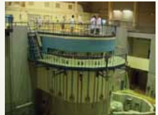
IRT-1 research reactor
