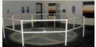
NIRR-1 reactor top
