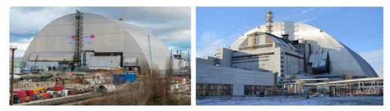
FIG. A-6. The New Safe Confinement over Unit 4 of the Chernobyl NPP (left, view from the construction site; right, view from Unit 3). The structure is 108 metres high, 162 metres long and 257 metres wide, and weighs about 36 000 tonnes. (Photos: Chernobyl NPP)
