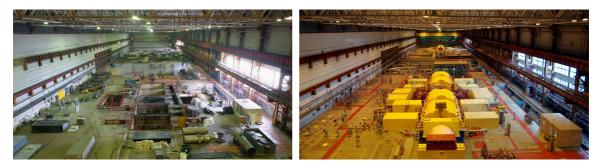
FIG. A-7. Dismantling activities at turbine halls of Units 1 (left) and 2 (right) of Lithuania's Ignalina NPP (Photos: Ignalina NPP).
