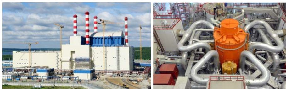
FIG. B-2. The BN-800 sodium cooled fast reactor started commercial operation on 31 October 2016. (Photos: Rosenergoatom)
