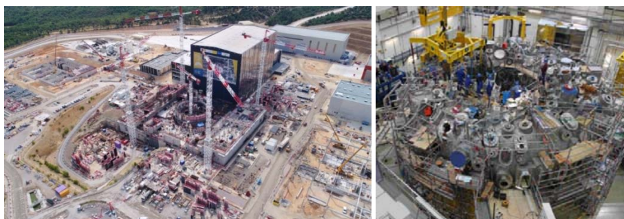
FIG. B-4. Left: ITER site in October 2017. (Photo: ITER IO). Right: Outside view of stellarator Wendelstein 7-X. (Photo: Max Planck Institute for Plasma Physics)
