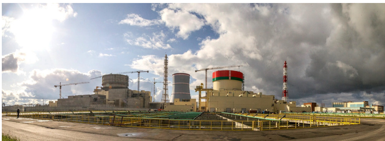
Ostrovets nuclear power plant, Belarus (Photo: Ministry of Energy, Belarus)
