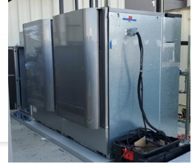
Bloom prototype 100 kW HTE system at INL Source: INL, 2022
