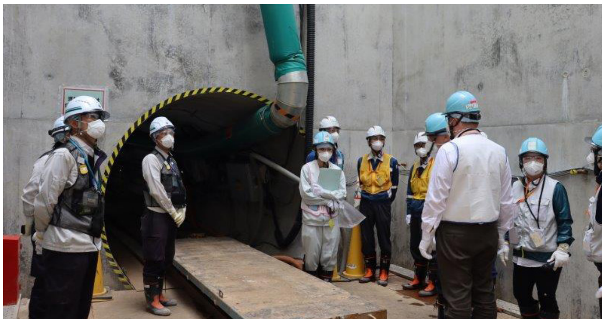
Figure 3.9. Inspection of the construction of the discharge tunnel
