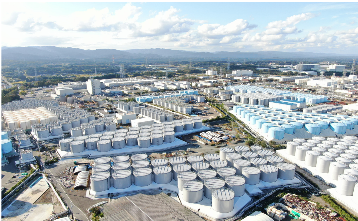
Figure 1.2. Storage tanks for contaminated water at FDNPS
