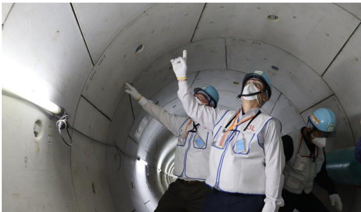
Figure 3.8. Pre-service inspection of ALPS discharge facility
